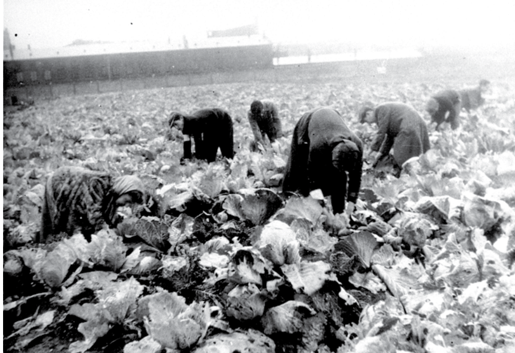
A garden on the site of Skra, the former sports stadium on Okopowa Street in the Warsaw ghetto in 1940.
