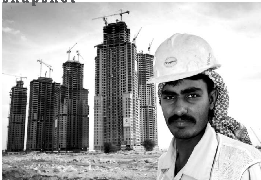
DUBAI, UNITED ARAB EMIRATES — A construction worker from Pakistan poses on a building site in Dubai on December 5, 2006. An estimated 20 percent of the world's cranes fill Dubai's skyline as this city of 1.4 million establishes itself as one of the great international tourist destinations. (Photo by Chris Jackson/Getty Images)
